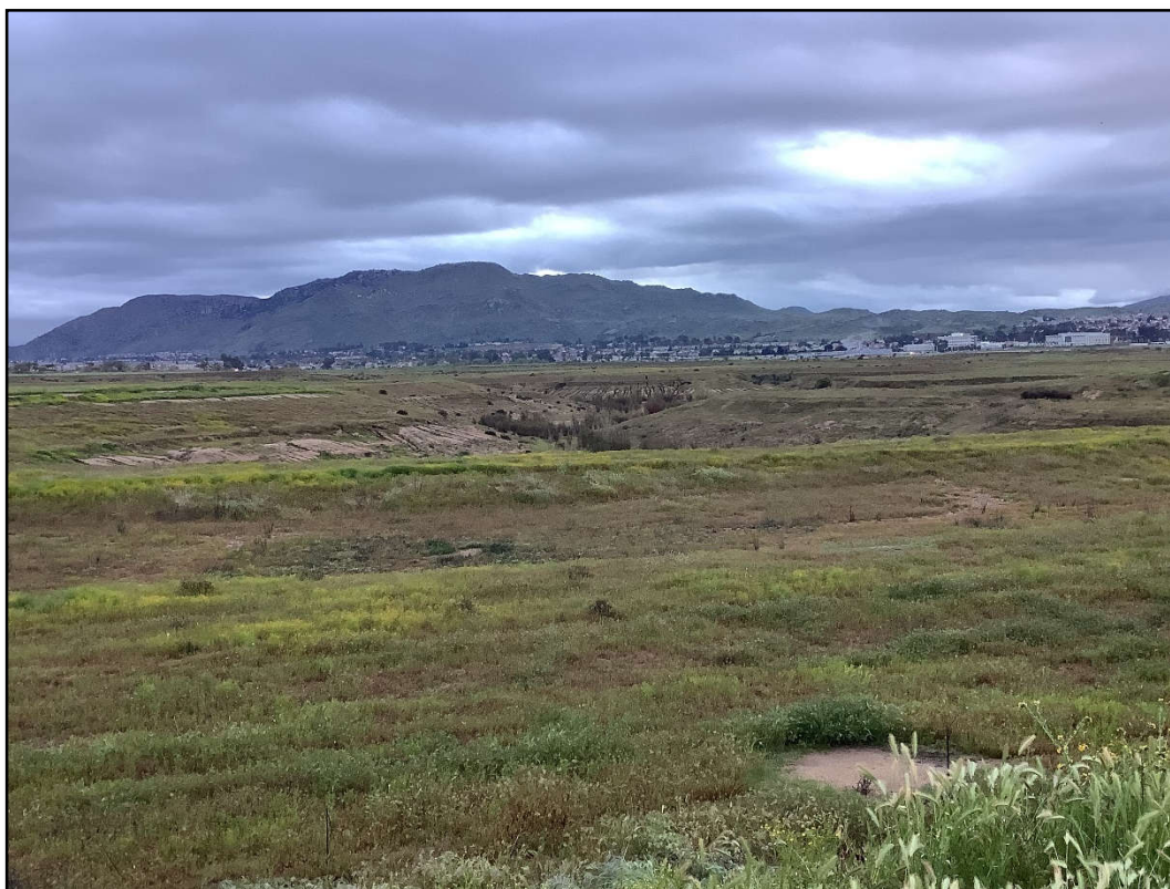
Photo 1: Facing east, overview of basin cuts.
