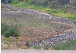
Figure 3: Gravel filled low-flow trench
