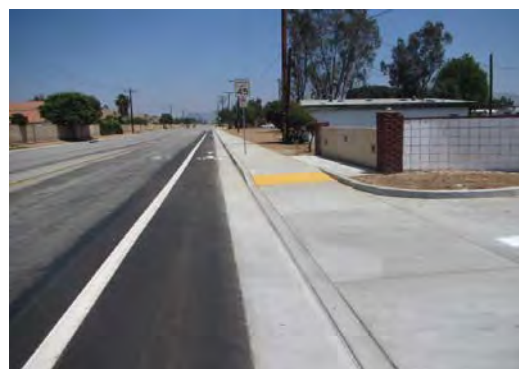
Pedestrian Ramp Improvements
