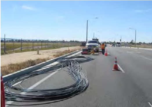
Citywide Fiber Optic Communications Expansion
