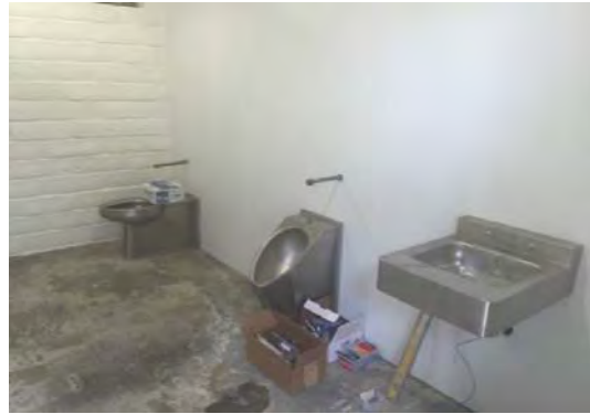
Park Restroom Renovations
