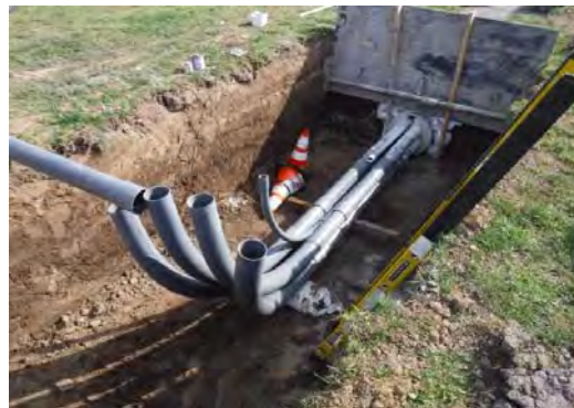
Feeder Line Trenching
