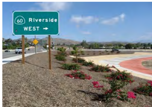
SR-60 / Nason Street Overcrossing Bridge (Landscape Establishment)
