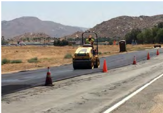
Pavement Rehabilitation Program
