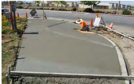
Pedestrian Ramp Improvements
