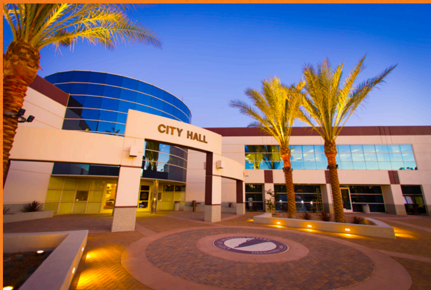
Civic Center Site Improvements (City Hall Exterior)
