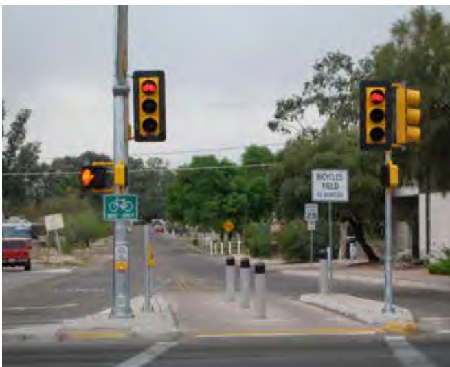
Bicycle signals - Tucson, AZ
