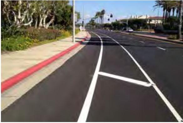
6B) Buffering repurposes extra space from travel lanes to provide more distance between cyclists and vehicular parking or traffic. Extra space converted to buffering should be diagonally striped so it is not mistaken as a travel lane - Huntington Beach, CA
