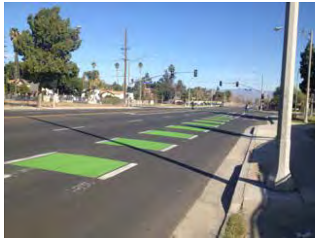
Green lane and merge zone - Riverside, CA
