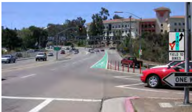
Green transition lane (Simulation with recommended signage) - College Boulevard at I-8, San Diego, CA
