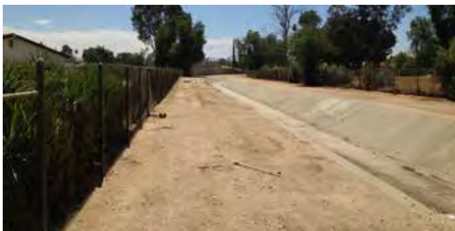
Typical flood control channel
