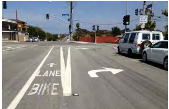
11B) Bicycle lane properly installed between through travel lane and right-turn-only lane - Huntington Beach, CA
