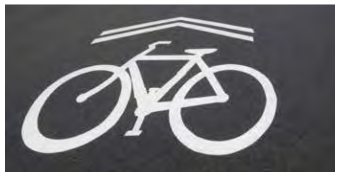
Shared lane marking (“Sharrow” or “SLM”)
