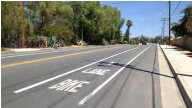
Bicycle lane - Indian Street
